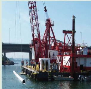
Ballard Diving is providing underwater inspection services. They are checking final grade on the installed pipelines and looking at side sewer piping, valves, bedding and trench configurations.
